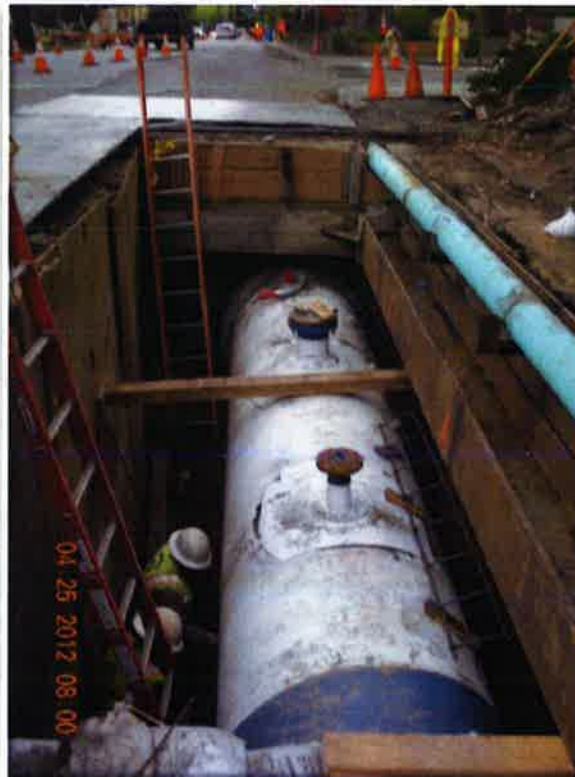
Crystal Springs Pipelines - # 3
