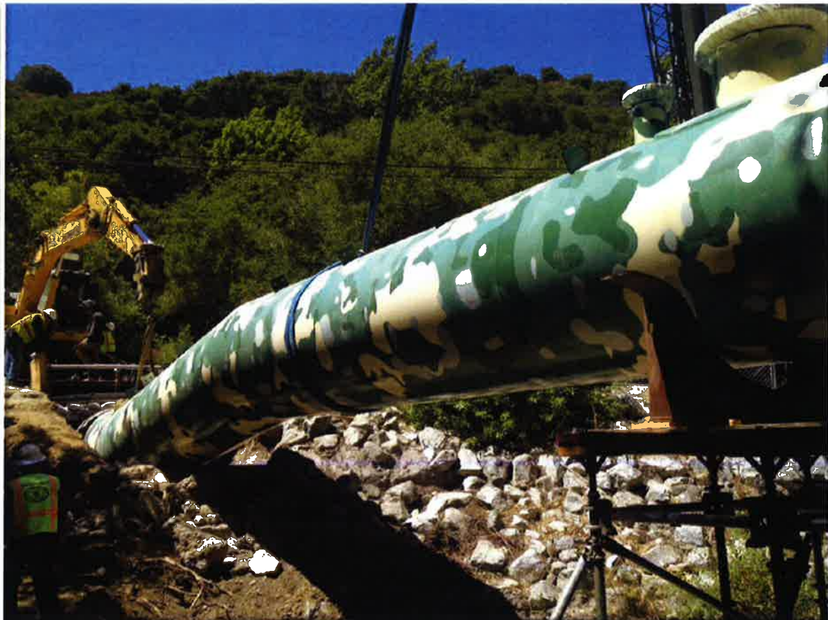
Crystal Springs Pipelines - # 1
