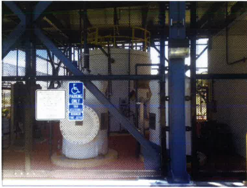
San Antonio Backup Pipeline - # 3
