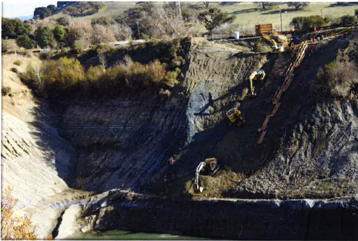
San Antonio Backup Pipeline - # 1
