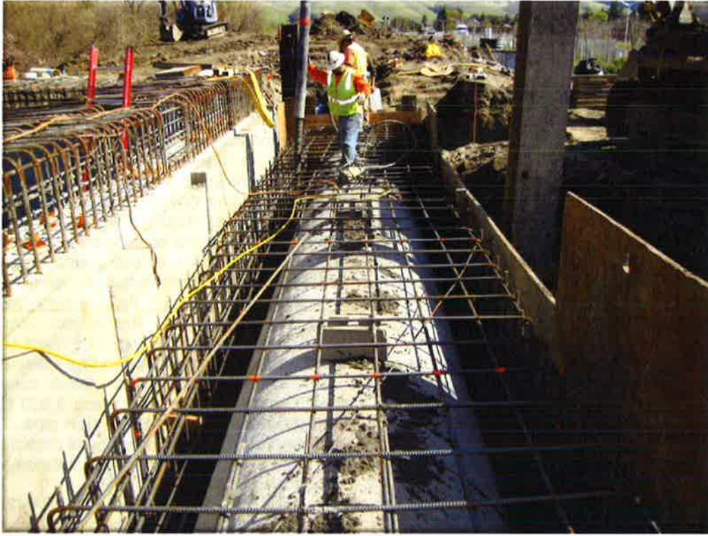
Bay Division Pipelines - # 2
