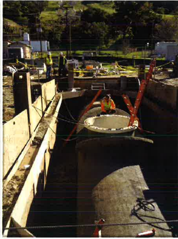
San Antonio Backup Pipeline - # 2
