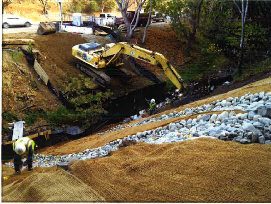
Crystal Springs Pipelines - # 2
